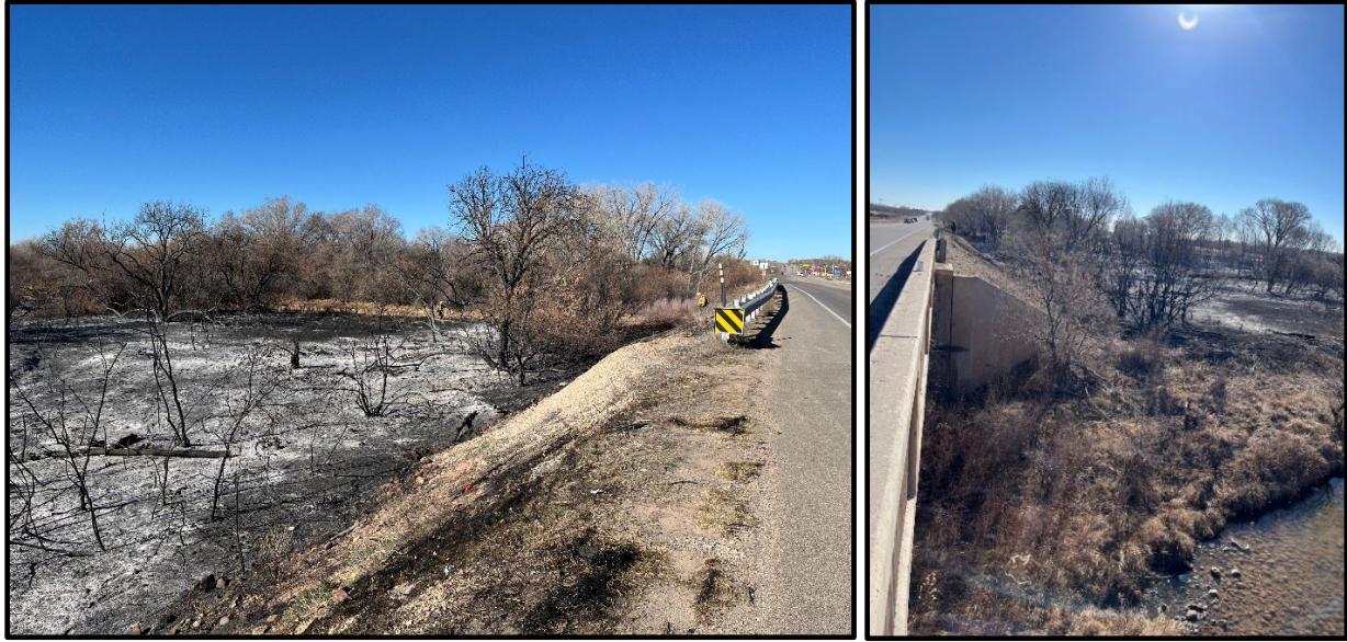
Figure 3: Left – View from the roadway looking toward the Uintah River bridge. Right – Looking east from the Uintah River bridge.
